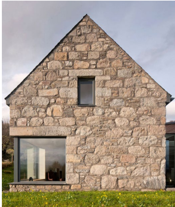
PREFERRED APPROPRIATE EXAMPLE OF LINTELS
