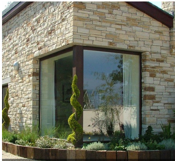
NOT PREFERRED UNAPPROPRIATE EXAMPLE OF LINTELS
