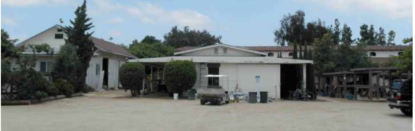
Figure 3.12 View looking east of all stables historic and non-historic
