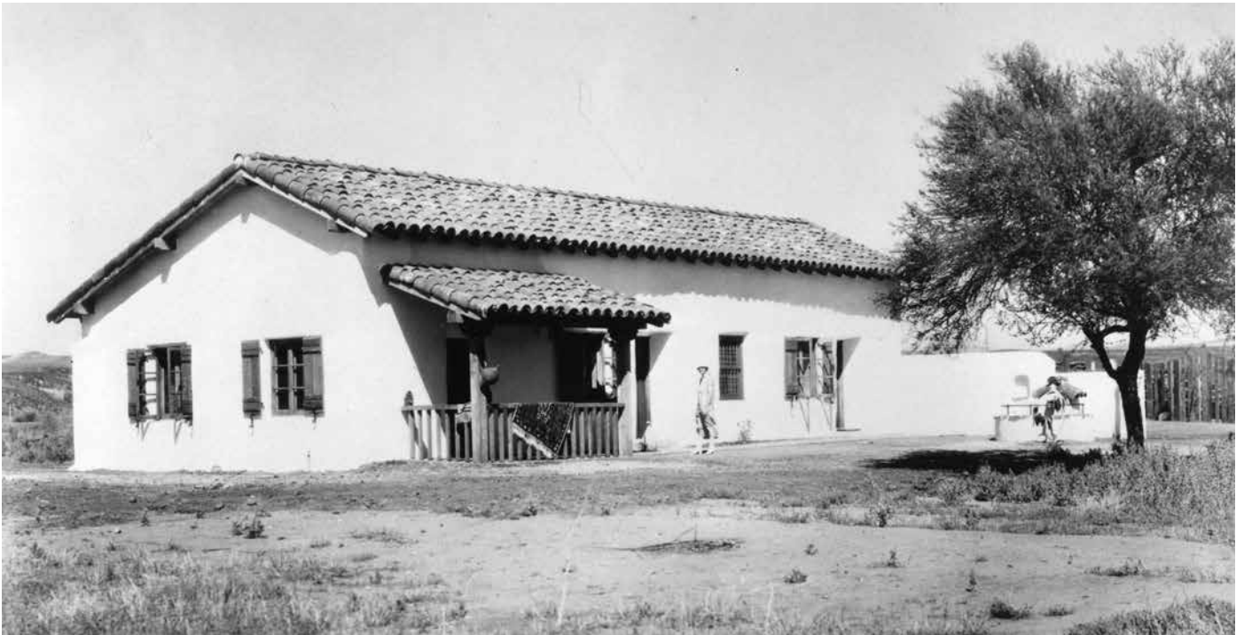
Figure 2.7 Completed Rehabilitation of Osuna Adobe #1
