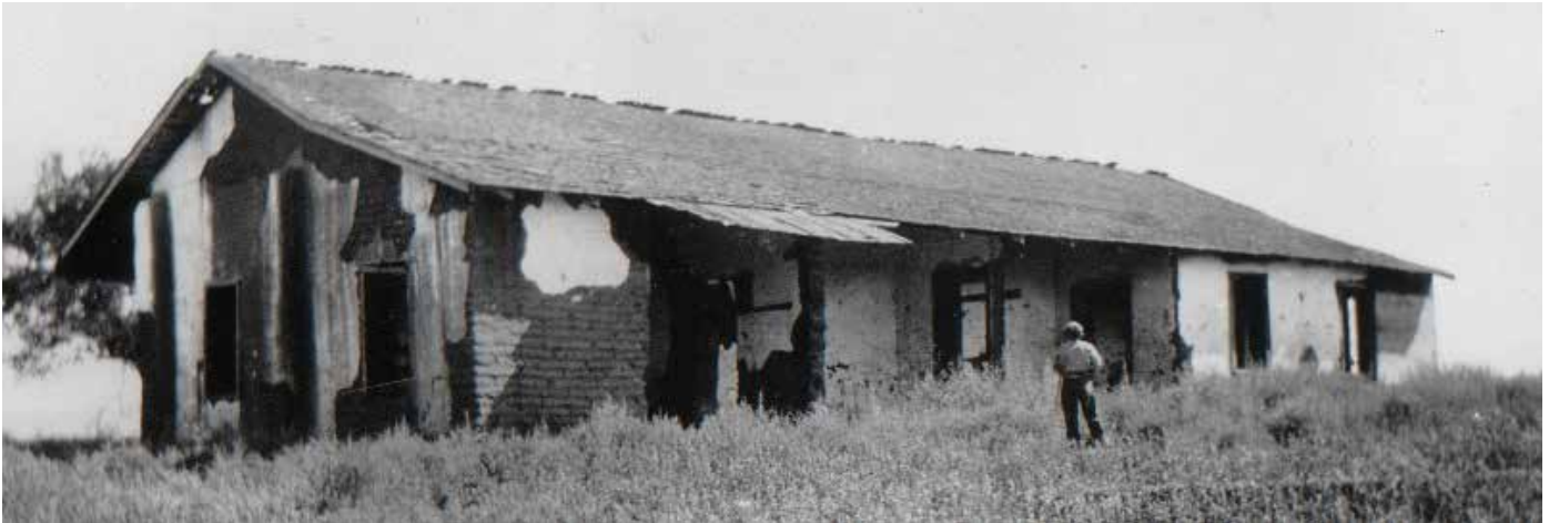
Figure 2.2 Remnant of the Osuna Period of Significance – Front elevation
