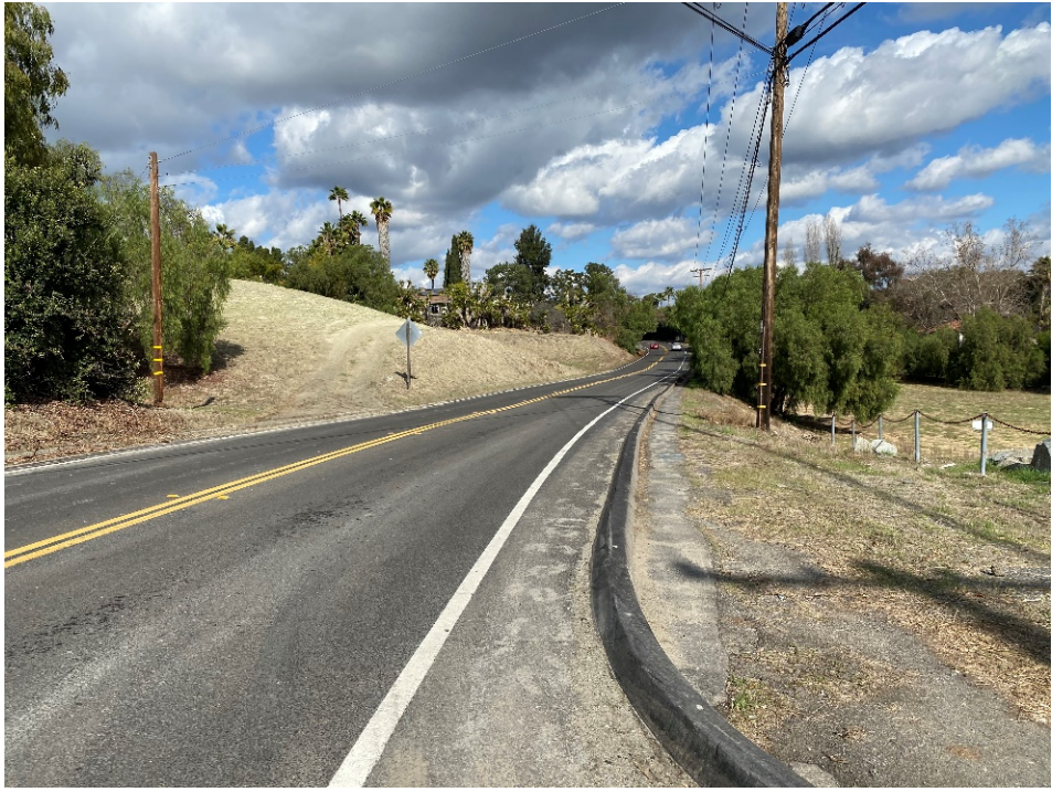
Rancho Santa Fe Road near Encinitas Blvd., Looking North
